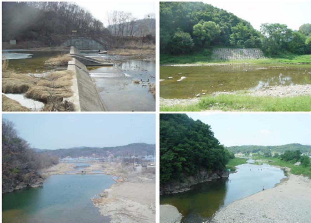
Figure 4.4 Gongreung 2 dam before (left) and after (right) the dam removal (KICT 2008)
