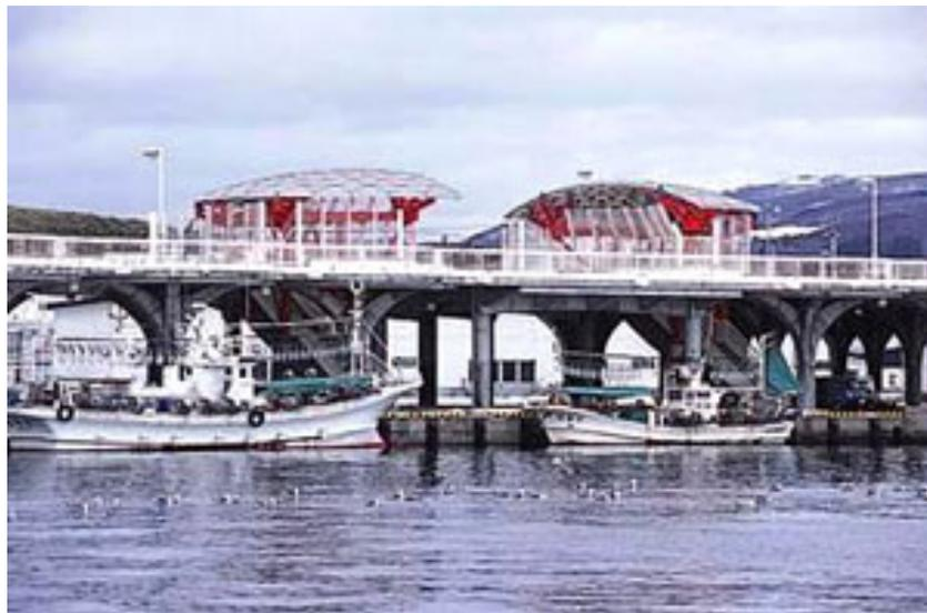
Photo 1.3 Tsunami refuge terrace at Aonae fishery port
