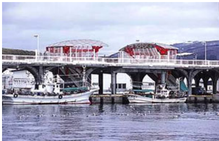
(a) Tsunami refuge terrace at Okushiri town Source: http://www.town.okushiri.lg.jp
