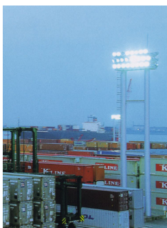
(c) Light tower in container terminal Source: Nagoya port terminal public corporation
