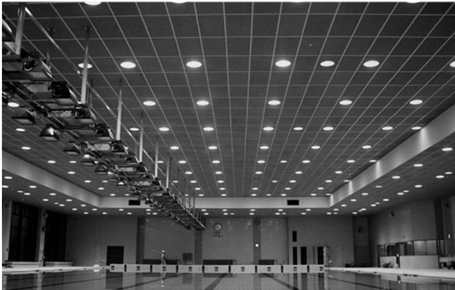
Fig. 1-2 Example as the absorbed sound material that was applied with the wall and ceiling of the Japan national sports science center.
