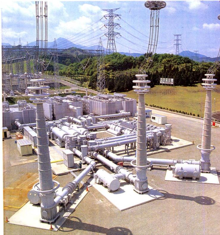
Fig.1.1 1000kV GIS and transformer for verification tests<sup>[9]</sup>.
