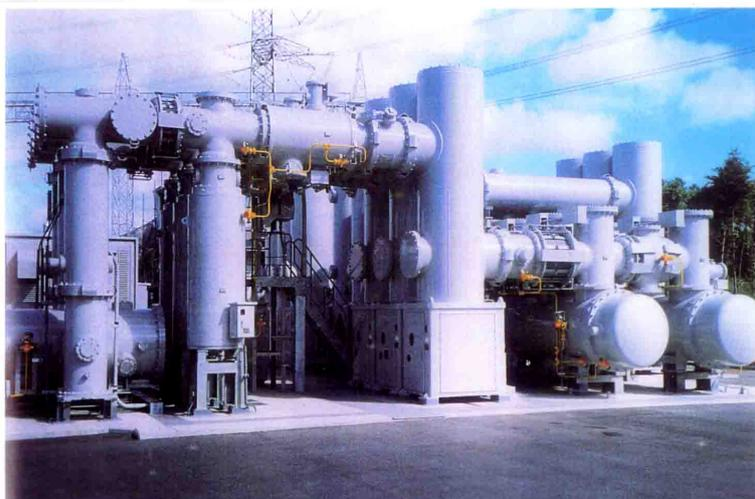
Fig.1.2 550kV GIS with 1 break GCB.
