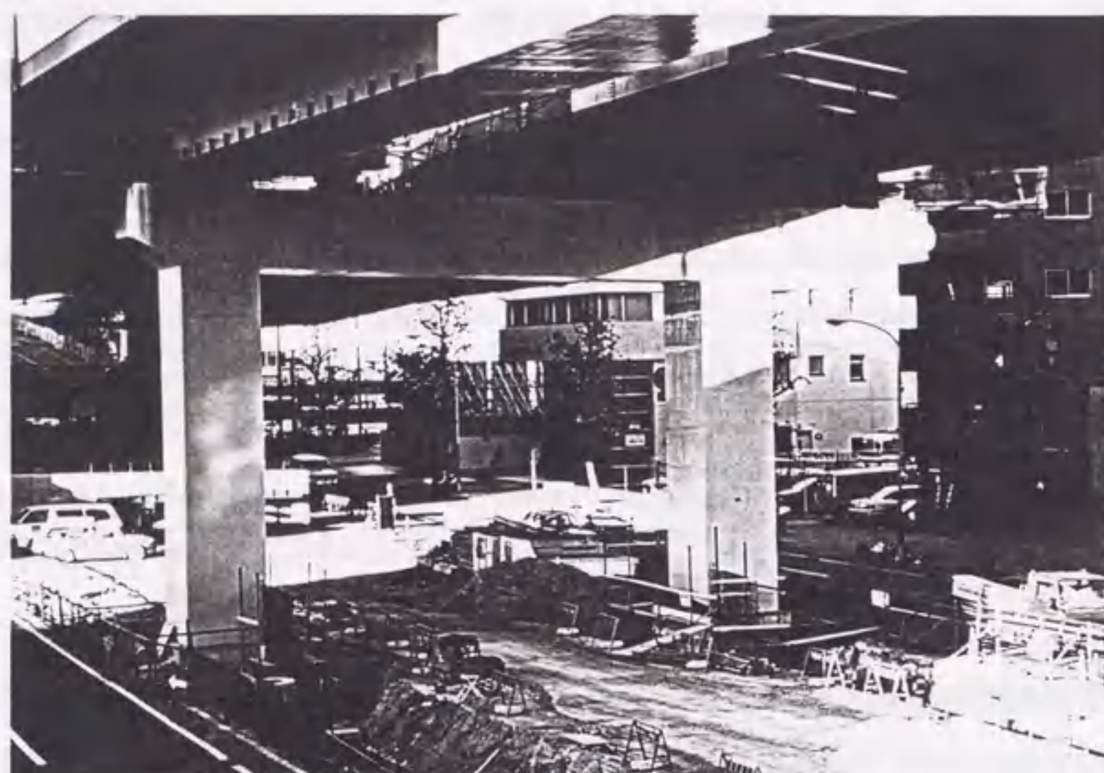
Fig. 1.2 Partially Concrete-Filled Steel Bridge Piers
