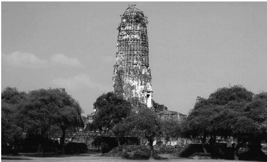
A ground-level view of the tower which symbolizes Mount Sumeru at Wat Phra Ram.
