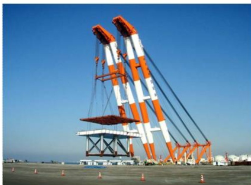
(c) Transport of steel jacket
