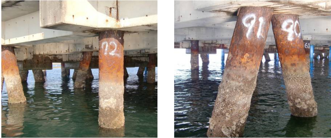
Fig. 1.1 Corrosion-damaged pipe piles at an offshore pier
