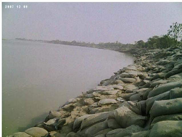
**Fig. A. 10** Jamuna River Right Bank Levee protection by geobags (Source: Field Investigation, 2007)
