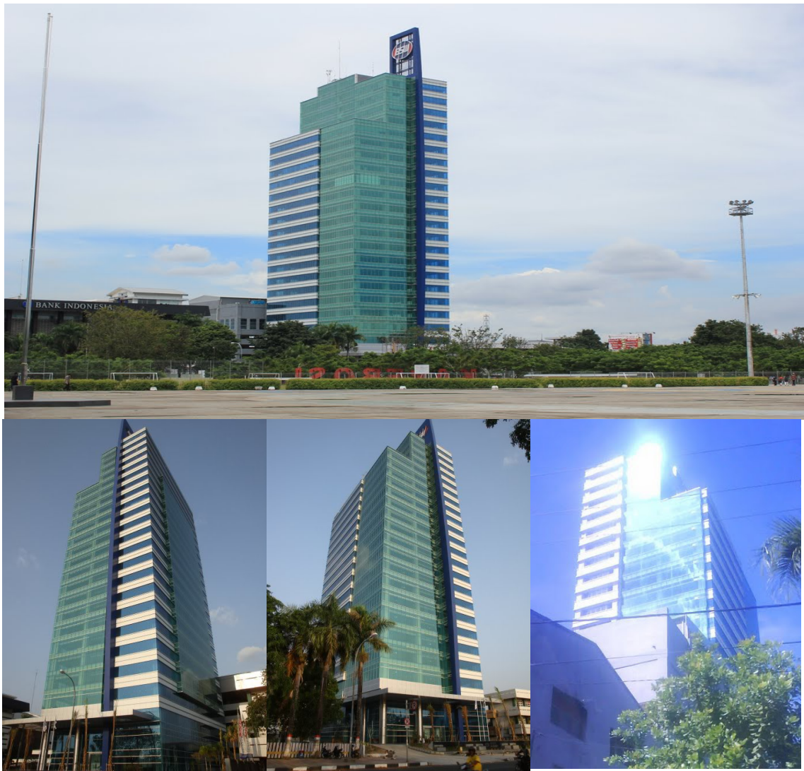
Figure 5.1-1. Views of “Menara Bosowa”
