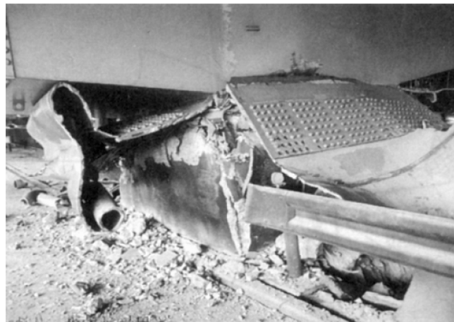
b) Ruptured steel bridge pier by cracks of corner weld
