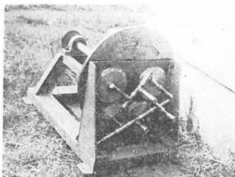
Photo. 6. A duplex switch for use at 1000 Mc/s. (just before installation)
