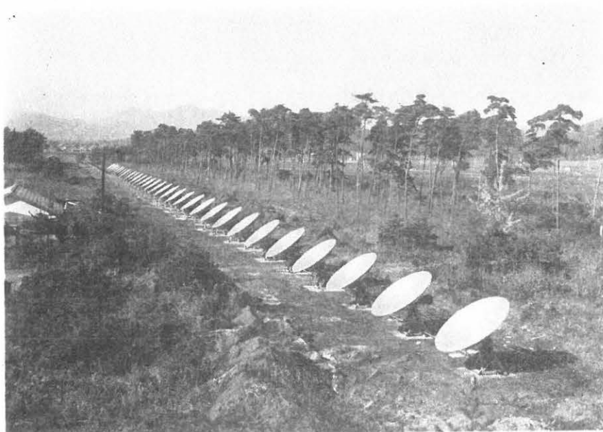
Fig. 2. A 3750-Mc/s compound interferometer under construction.
