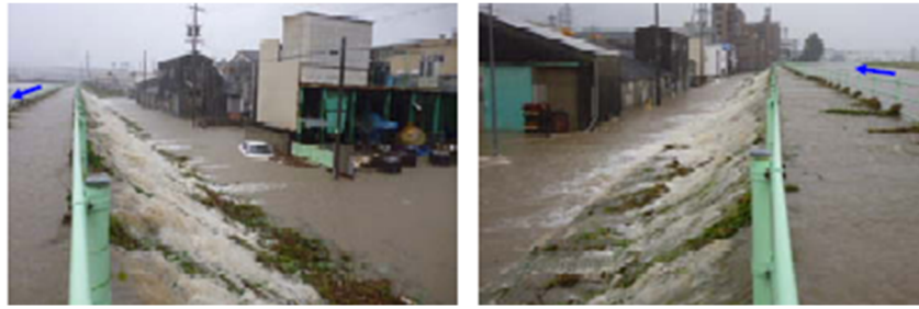
Figure 5-5 Levee overflow in the Hatta river and consequent damages to private assets (Thomas et al, 2014)
