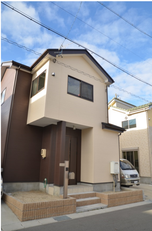
Figure 5-22 houses constructed after 2012 with first floor inhabited, structural enhancements for urban flood or small-scale flood (detail, January 2014)
