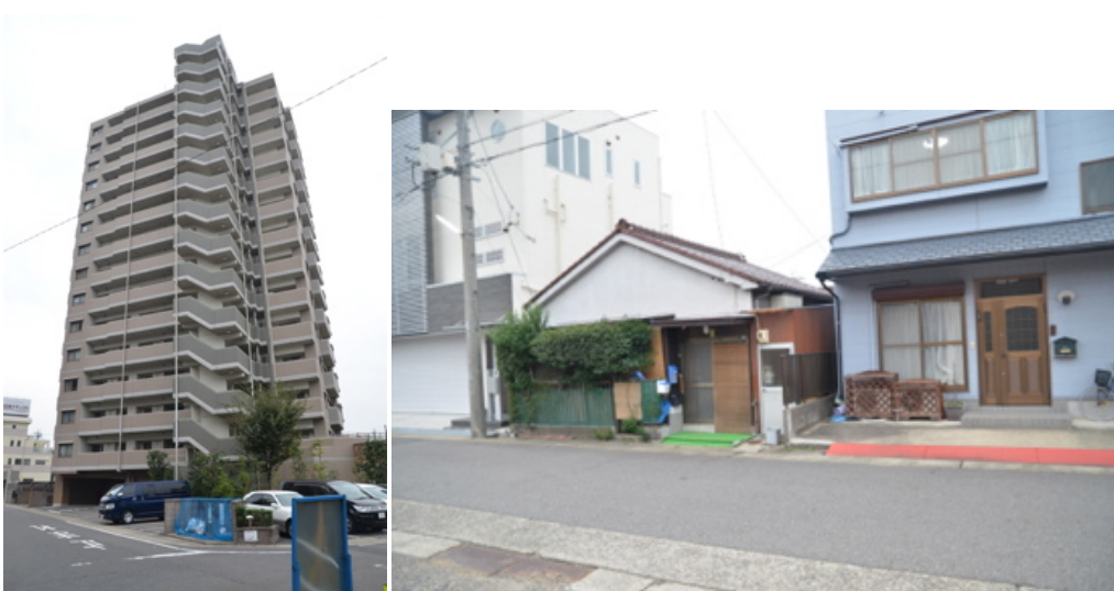
Figure 3-23 (left) type A building protection type 3 (right) type C building no protection (type 1)
