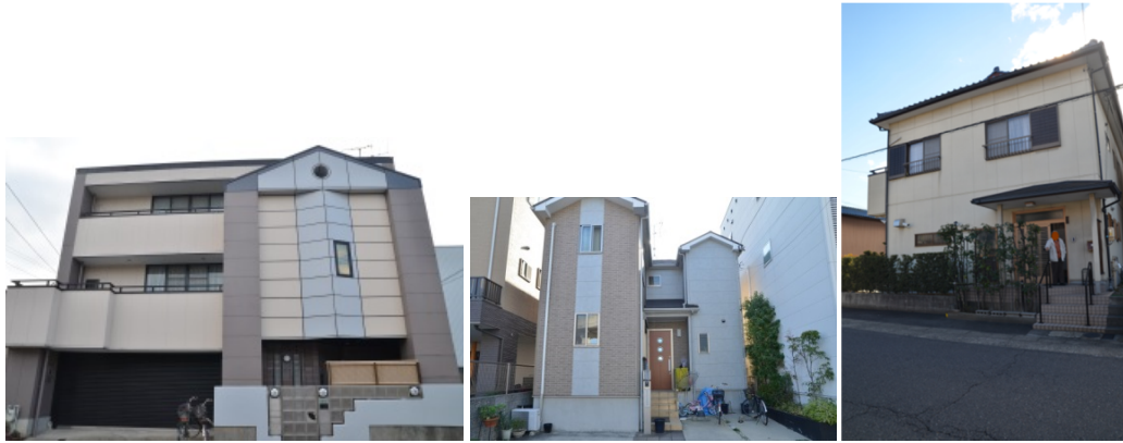
Figure 3-24 inherent problem to protection type 2 (0-1,5m) done on type B buildings
