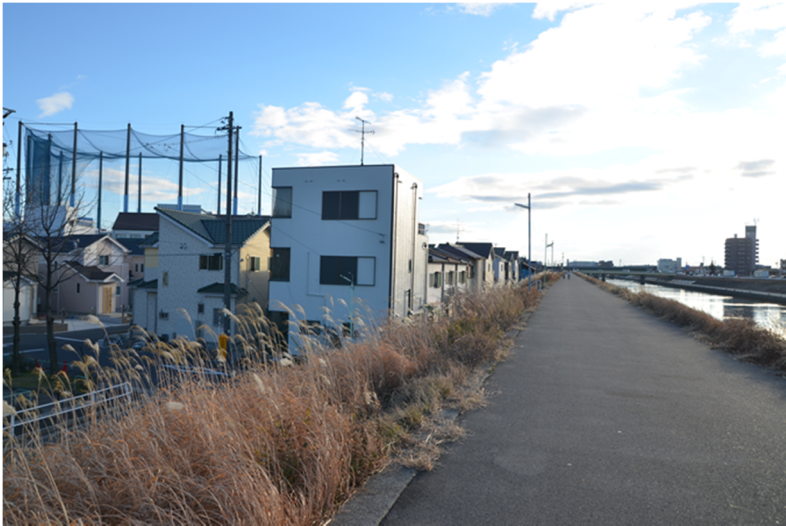
Figure 5-21 houses constructed after 2012 with first floor inhabited (January 2014)
