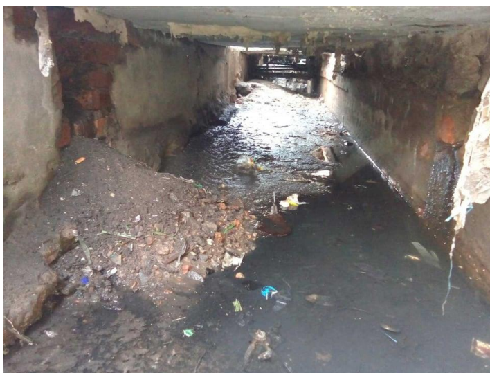
Figure 3.2 Sediment in the drain (source-DWMA Latha)
