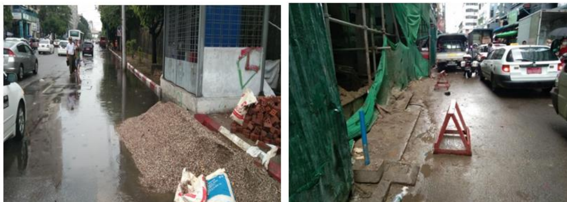
Figure 7.11 Construction materials, gravel and sand at the rear of drainage throats (source-DWA Latha)
