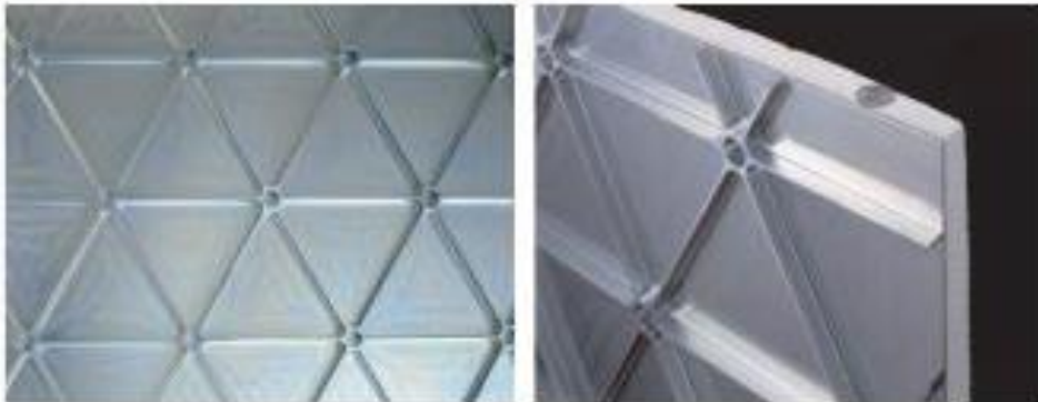
Fig.1.1-3 Isogrid structure [12]
