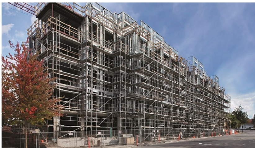
Fig1.2 Mid-Rise Construction with Cold-formed steel structure [1.9]
