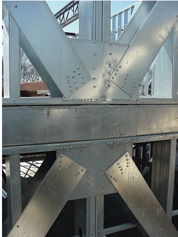
Fig 1.1 screw connections of Cold-formed steel structure [1.8]
