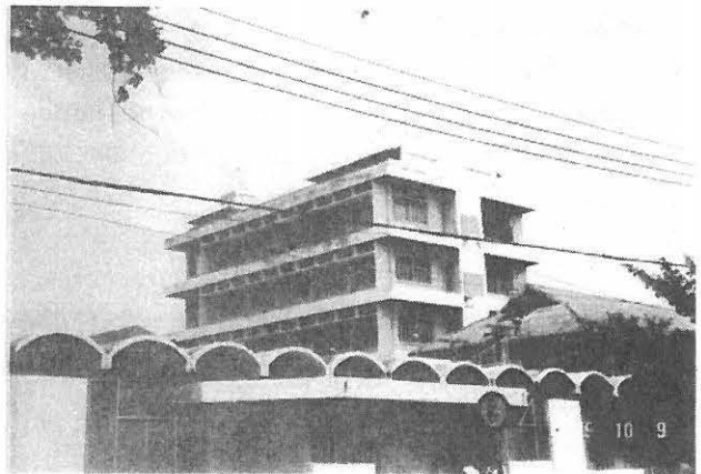
Fig.1 The exterior of the building of the Department of Electrical Engineering, Chulalongkorn University.
