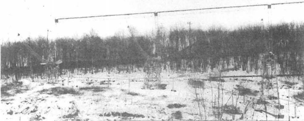
Figure 2. UHF cylindrical parabolic reflector at Sugadaira.
