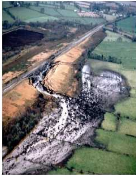
Photo 2. 2 Failure on Grand Canal embankment constructed on peat (Pigott et al. 1992)
