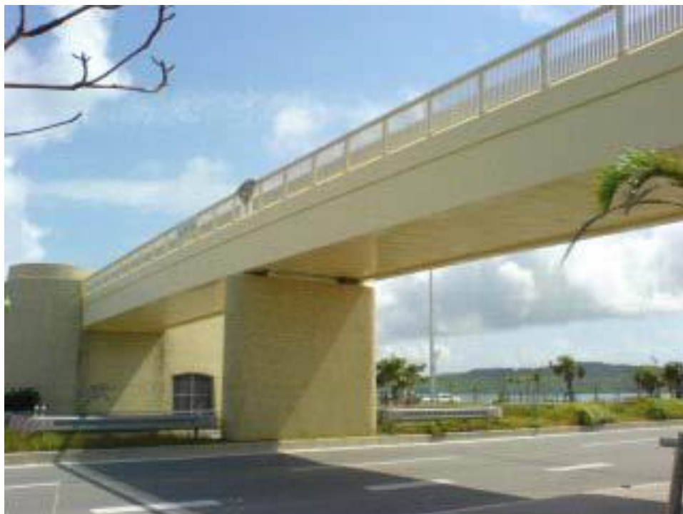
Figure 1.5: FRP pedestrian bridge, Okinawa, Japan (Courtesy: Dr. Itaru Nishizaki)
