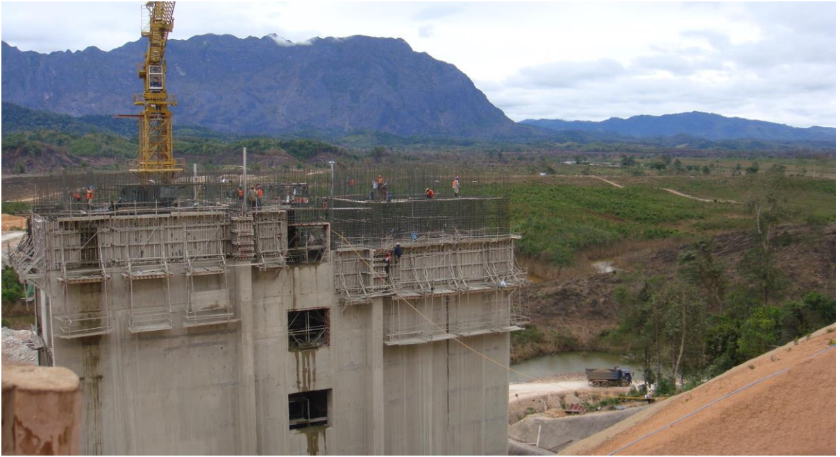
Photo 3-1A: Construction of THXP Source: Field survey, 2011
