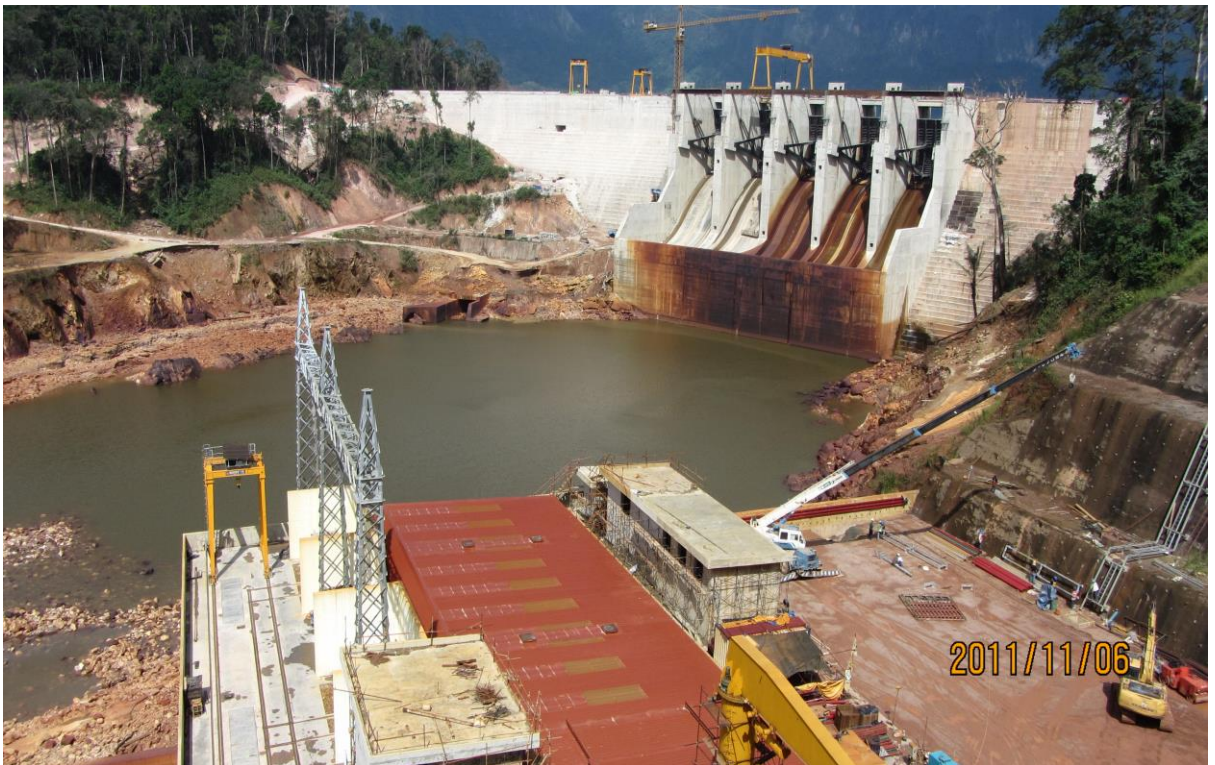
Photo 3-1B: Construction of THXP Source: Field survey, 2011
