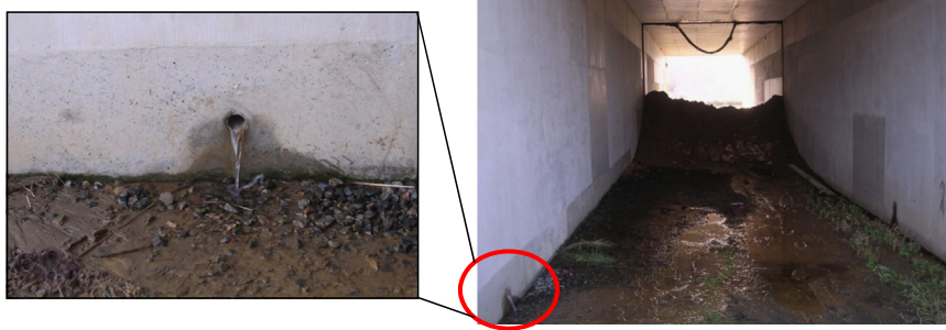
Fig. 26. Water outflow seen in a box culvert of a highway embankment on clayey ground affected by the Mid Niigata Prefecture Earthquake in 2004. (The earthquake occurred on 23 October 2004. These photographs were taken on 5 November 2004).
