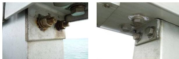
(a) 21 Years of service (b) 18 Years of service Fig. 1 Typical galvanic corrosion on guiderails in Okinawa 2013
