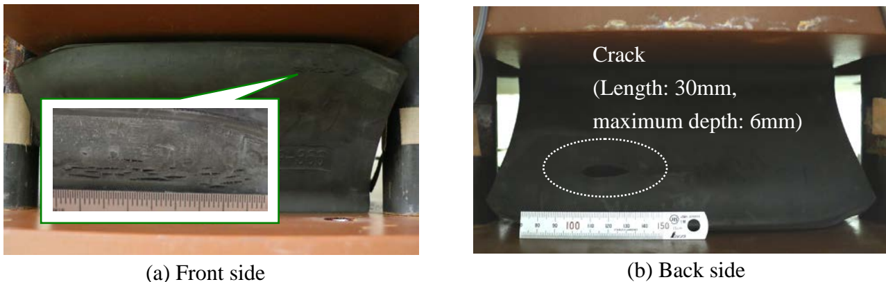
Figure 6: Cracks of bearing specimen
