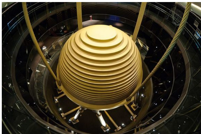
Fig.1.1: Picture of dynamic vibration absorber of Taipei 101 [3]
