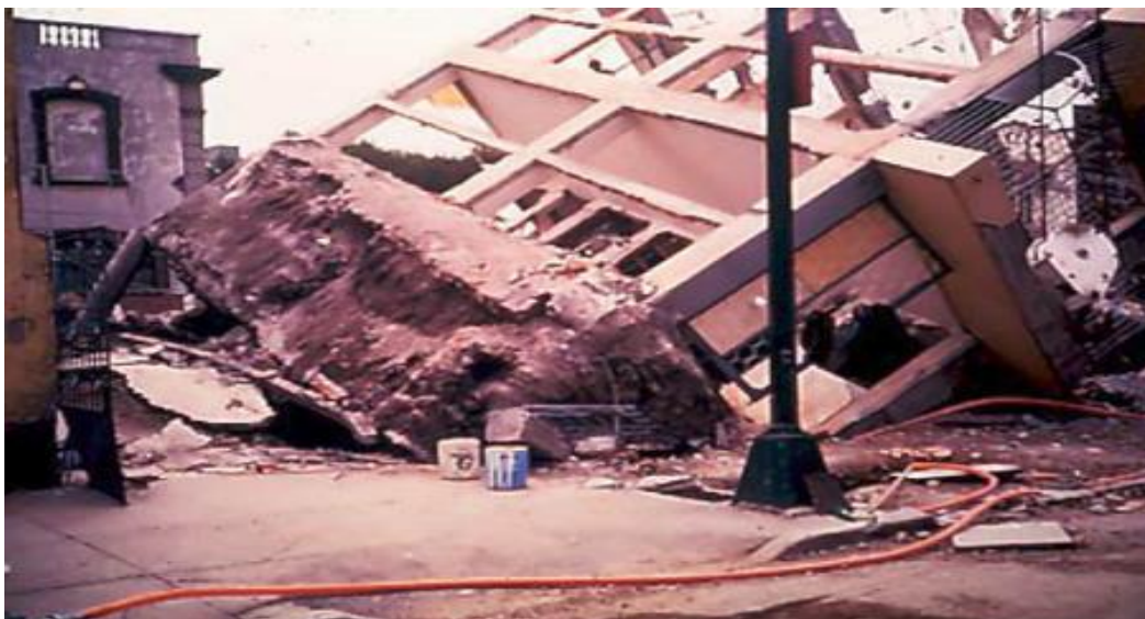
Fig. 5.1 Mexico Apartment (Earthquake 1985)
