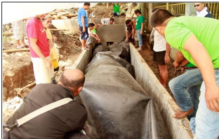
Figure 6.2 The 1st HDPED installed at the Biogas Training
