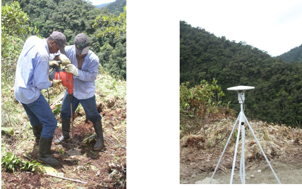
Figure 13. Shallow-drilled braced monument (ANCH station).
