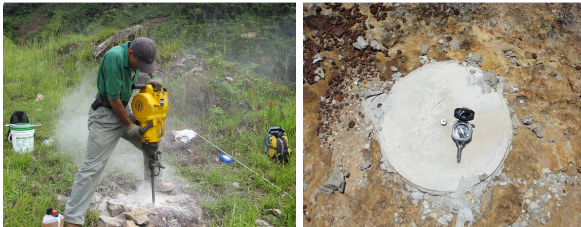
Figure 15. Field station installed on bedrock.
