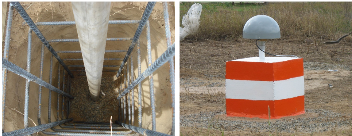
Figure 12. Reinforced concrete pillar (ALPA station).
