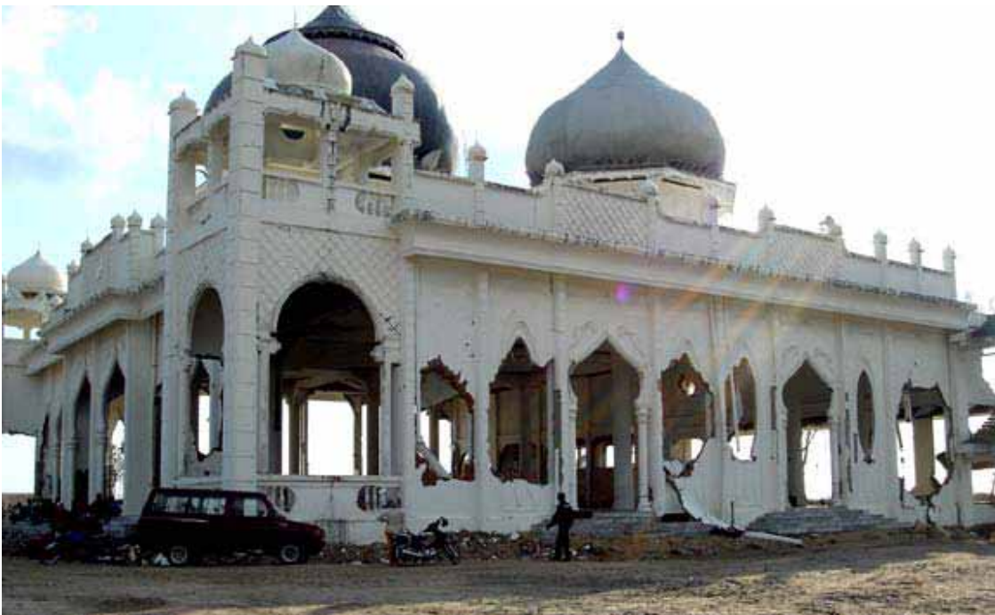
Figure 8: The mosque in Lhok Nga that was affected by tsunami waves.
