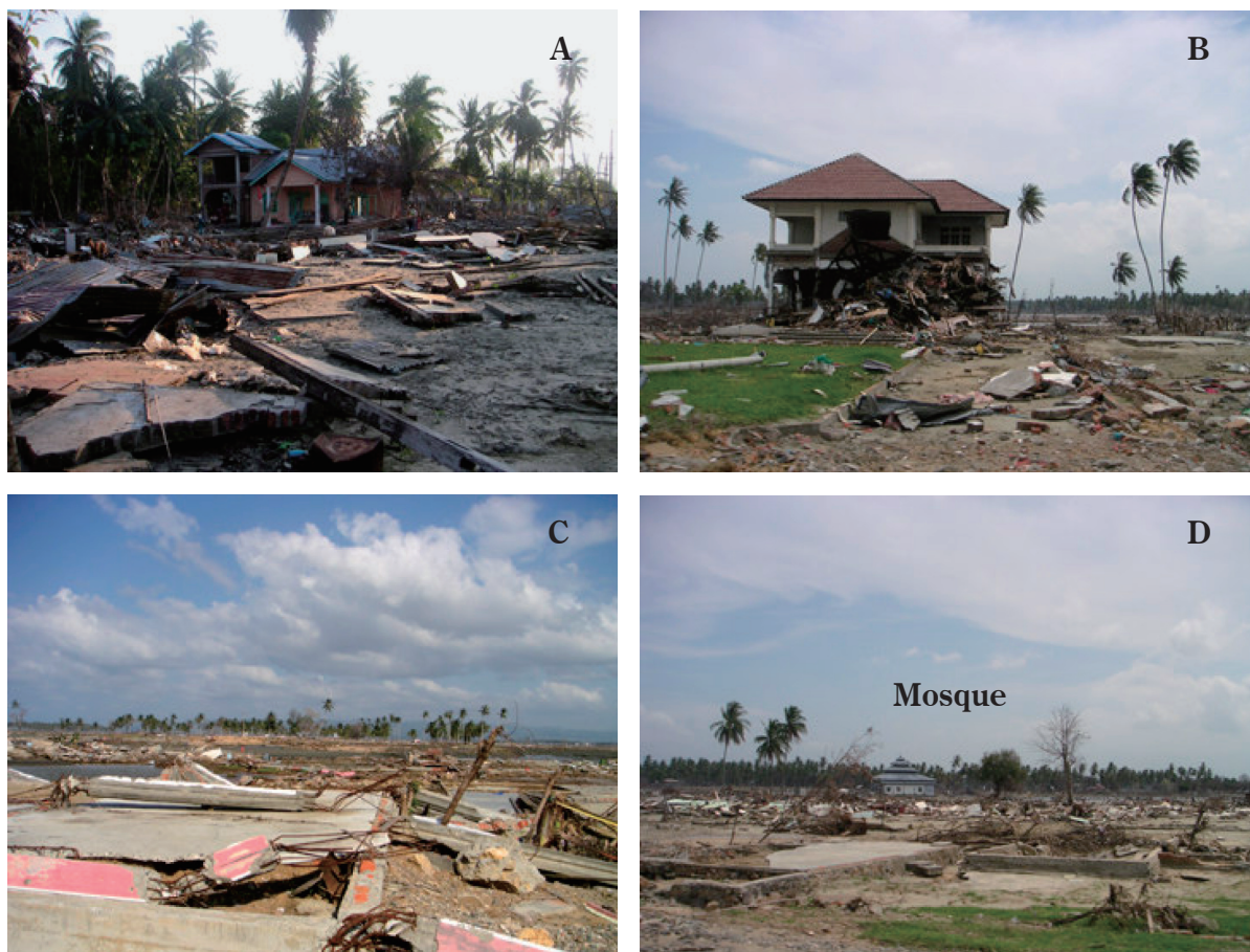
Figure 5: Photos showing damages from tsunami outside of the city of Aceh. Clockwise, a house in Krueng Raya about 100m away from the shore (A), 2-storey concrete house in Aceh Besar (B); totally destroyed community around a mosque in Aceh Besar (D); and remains of the house in Aceh Besar (C), where the similar directions of the bent columns along S16E can be noted.
