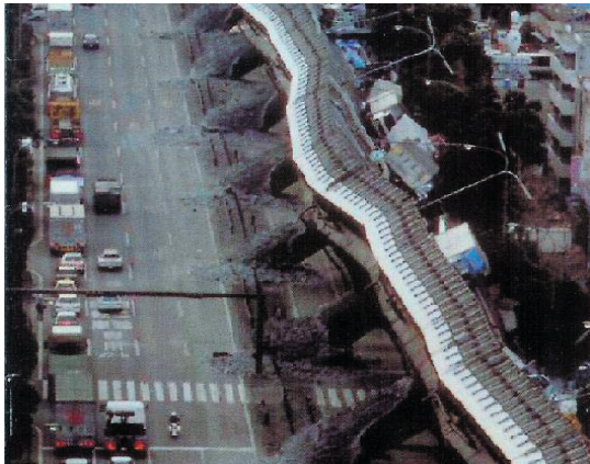
Figure 1. Hanshin highway was ruined after big earthquake in Kobe
