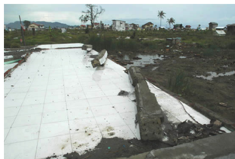
Fig. 8. Fallen columns indicating run-up tsunami direction
