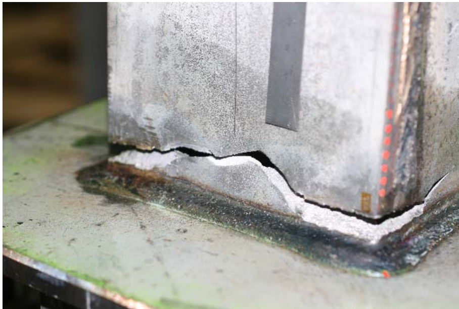
c) Crack through flange ( N=18.5 )
